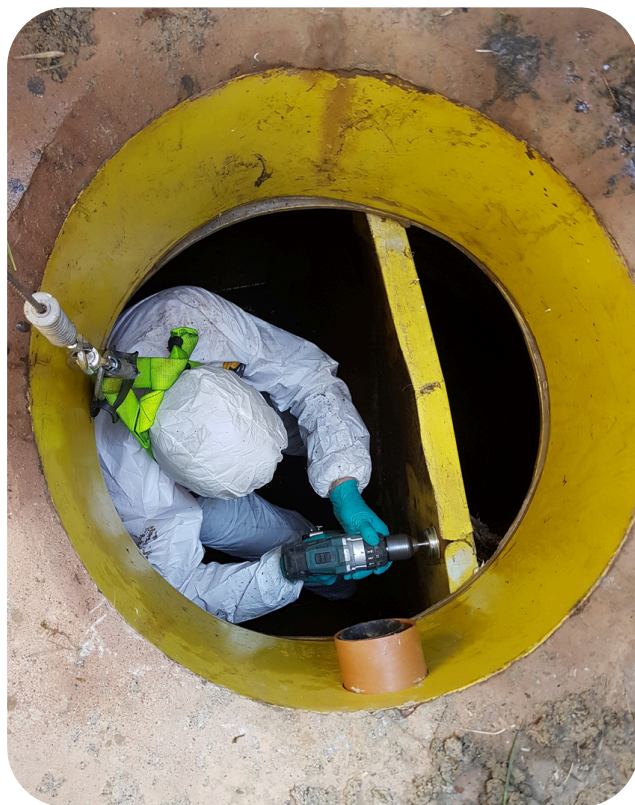
Above: Structural GRP repair through confined space entry
