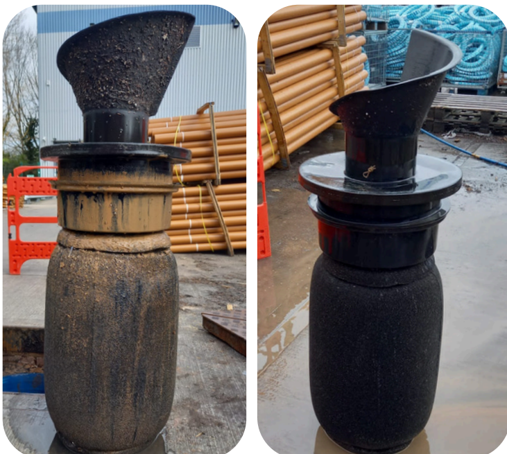
Below: Coalescer filter refurbished and reset
