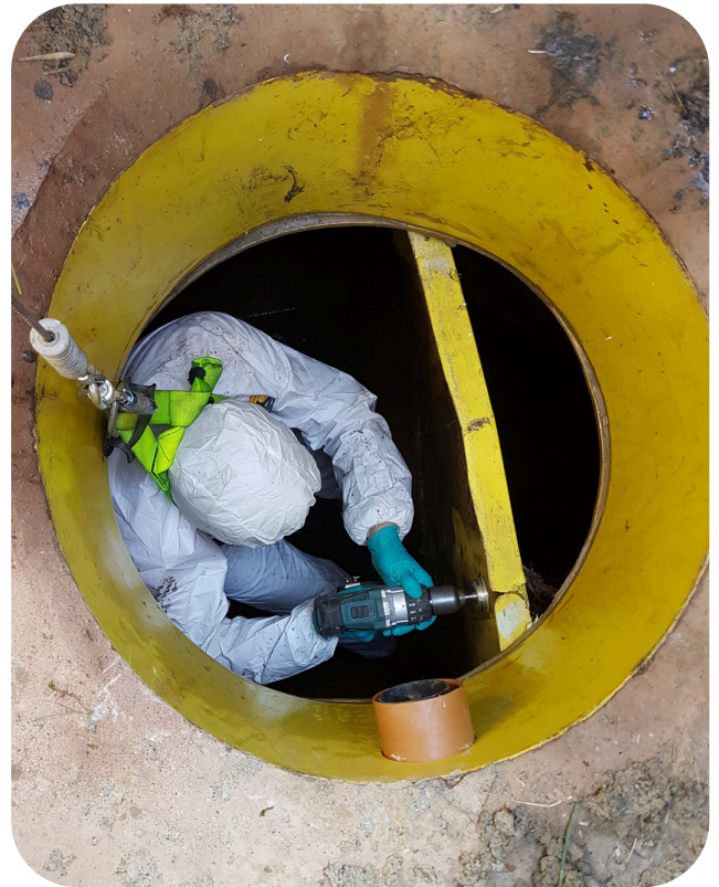
Above: Structural GRP repair through confined space entry
